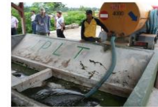
Sludge tanker disposing of liquid waste at a sludge treatment facility
